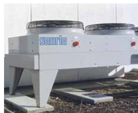
Heat exchanger of a glycol cooler
